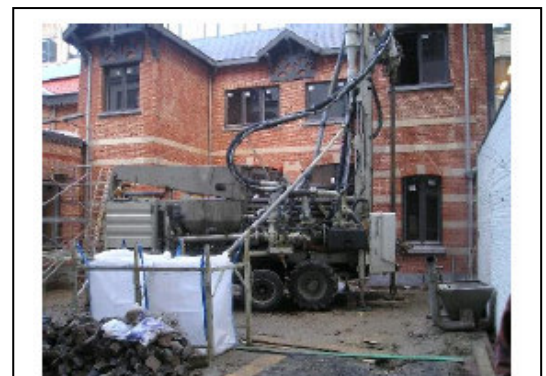
Drilling for BHE in the courtyard
